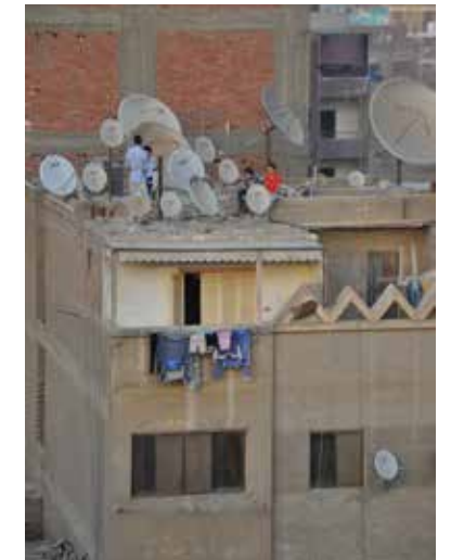
Figure 4.31 Installing a satellite dish
