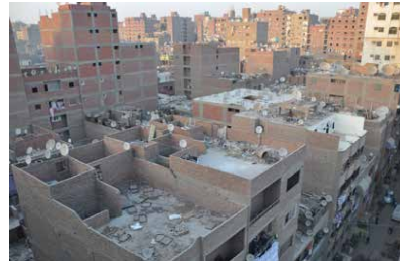
Figure 4.30 Rooftops in Ard El Lewa
